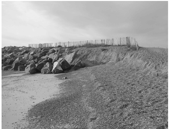
Figure 3: Scouring of the sea wall.
