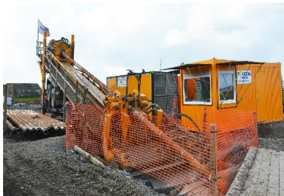
Drilling rig in place
