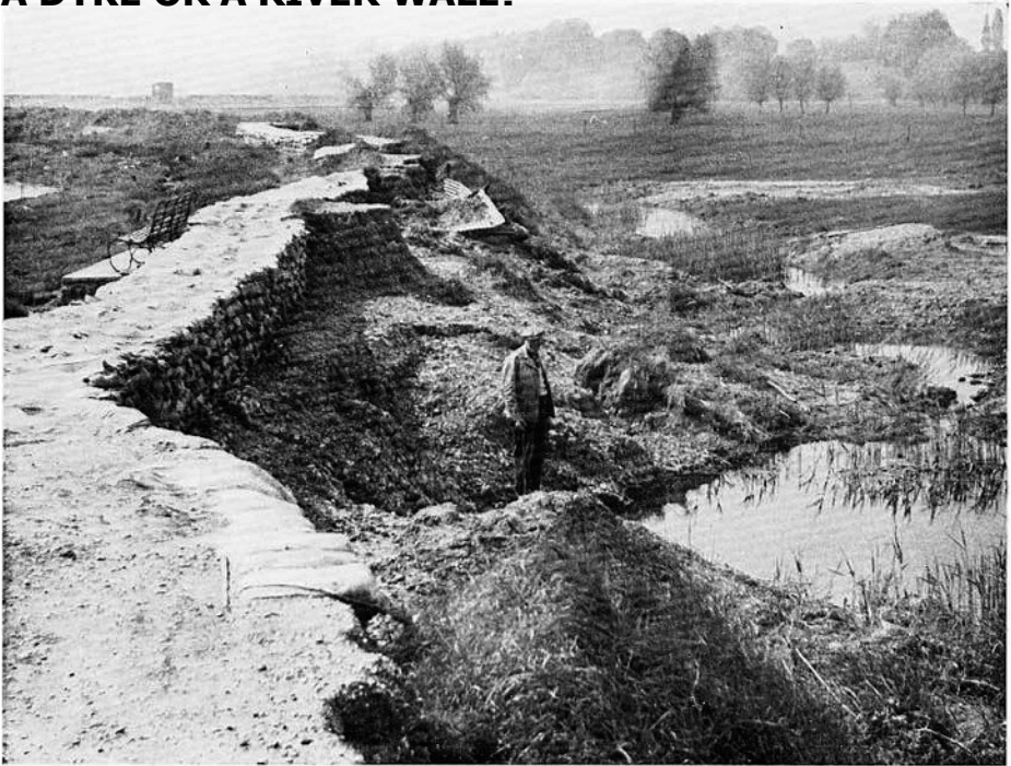
1962 temporary repairs to the Deben levees at Woodbridge.
