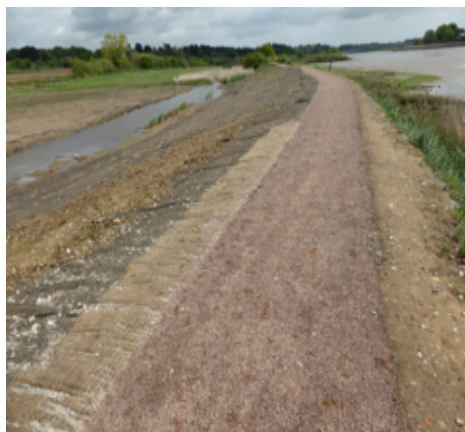
Geogrid with compacted crushed concrete
