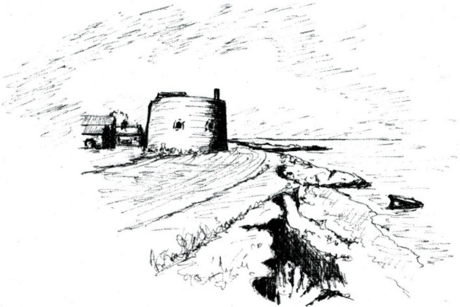
EROSION at BAUSDSEY MARTELLO TOWER.
