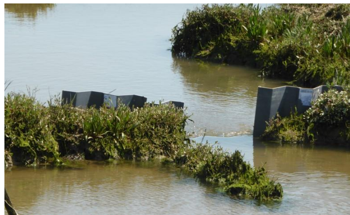
b) Sill created by sheet piling
