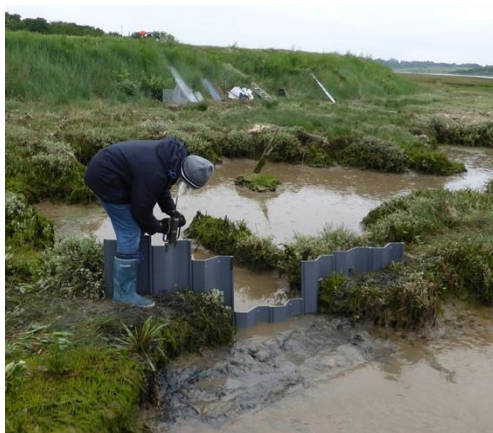
a) Installing the sheet piling
