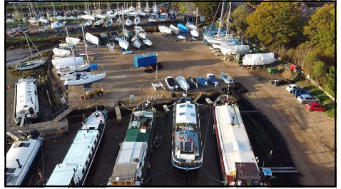
Aerial views of the new hard standing areas at Robertsons Boatyard.
